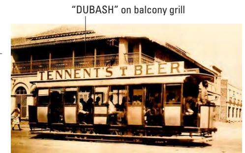
Cowasjee & Sons office behind trolley
