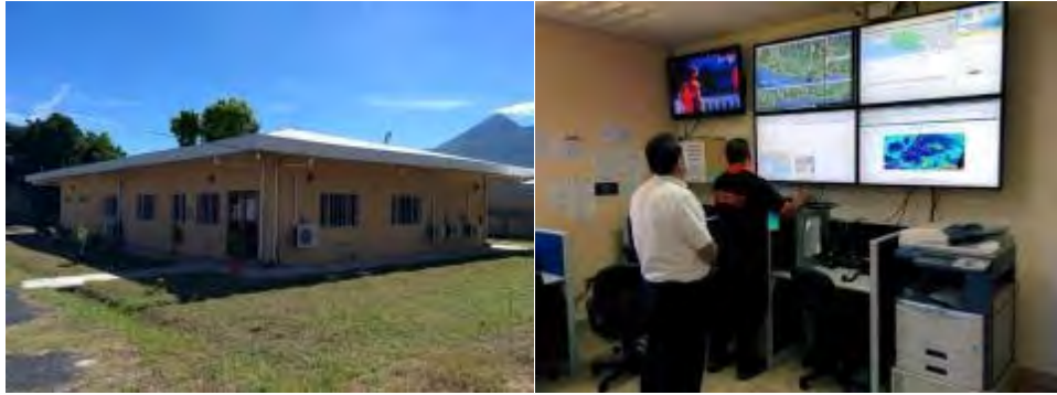
Figure 2.2.18 DGPC Emergency Operation Center, Facility Whole View (Left), Inner View (Right)
