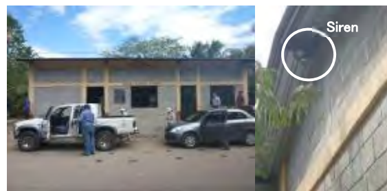
Figure 2.6.18 Evacuation Shelter (Community Center) and a Siren at Cedeño (Marcovia)
