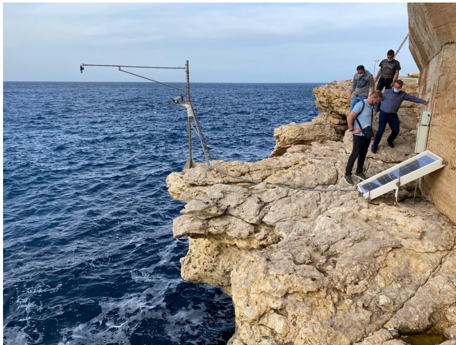
Figure 6: visit to IDSL-34 before the exercise, for maintenance intervention.
