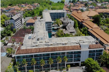
Hotel Roof Top for Vertical Evacuation
