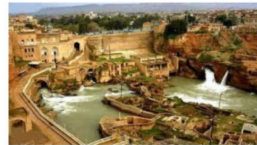
Water Structures –shoshtar –khuzestan
