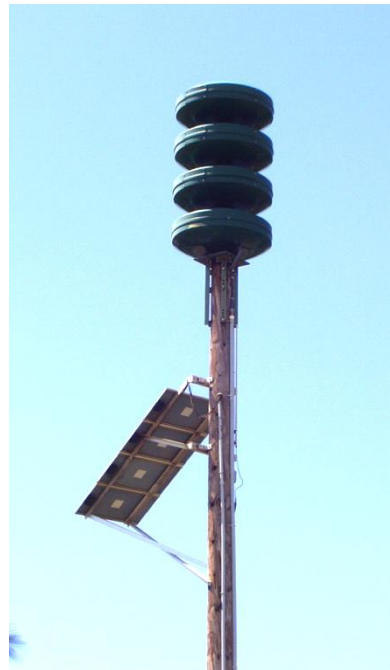
Figure S.58. Left. An empty propane tank and stick is used to sound the alert, Savaia, Samoa. Right. Omnidirectional sirens, with solar power backup, are used in Hawaii, USA. Photos courtesy of ITIC.
