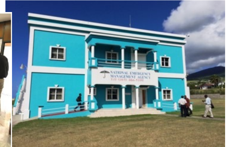
St. Kitts Emergency Operations Center
