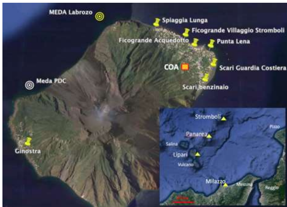
Figure 25. Position of the COA and the Acoustic Alert (siren) system used to warn population on the possible occurrence of a tsunami.
