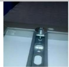
Please, note the position of the sliding nuts when blocked in the final position, they must be horizontal in respect to the bars to avoid to exit.
