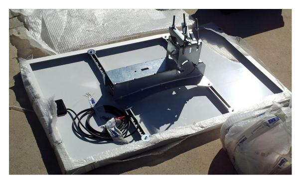
Pay attention to the wire that must not be pulled too much to avoid the removal of the contact with the electrical connections of the solar panel.
