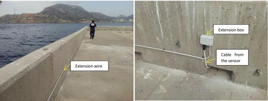
JRC provides the extension cable; this cable is planned to resist to outside conditions. It is however better to consider the installation of a plastic tube to protect it from direct sun exposure.
