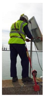
Once the mounting structure is completed, it is possible to fix the solar panel on the top of the pole. To facilitate the mounting of the solar panel it is possible to lower the pole to a more convenient position, fix the solar panel and position it at the correct vertical angle, then rise back the pole to its final position, including the right horizontal inclination (normally toward south).
