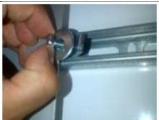
Insert the bolt with the washer positioning the sliding nut inside the bars. Below a detail of the sliding nut. Be careful to position the nut in the direction of closing otherwise it will not fix
