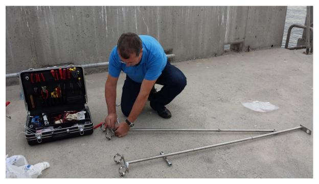
Once the installation of the arm is performed, it can be fixed to the pole using the screws. At this point it is possible to include the sensor and fix the sensor cable using 3 or 4 cable ties (or tie-wraps) along the horizontal part.
