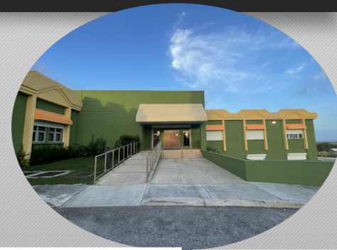
Image Showing the BMS.
