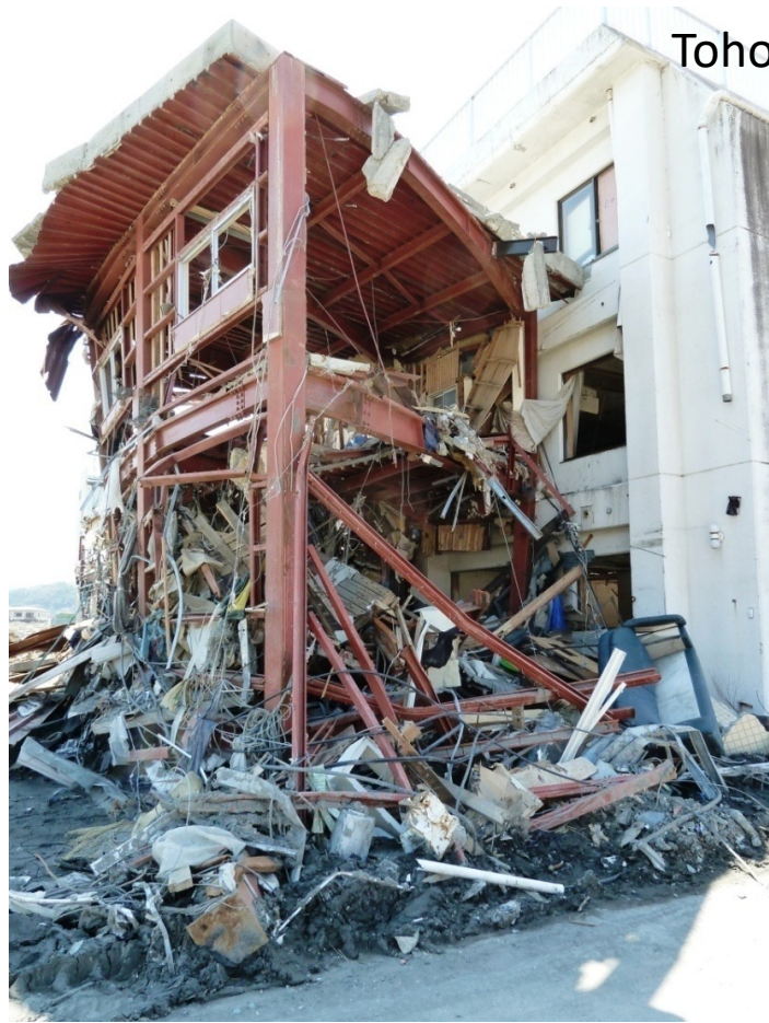
Three-Story Steel MRF collapsed and pushed into concrete building
