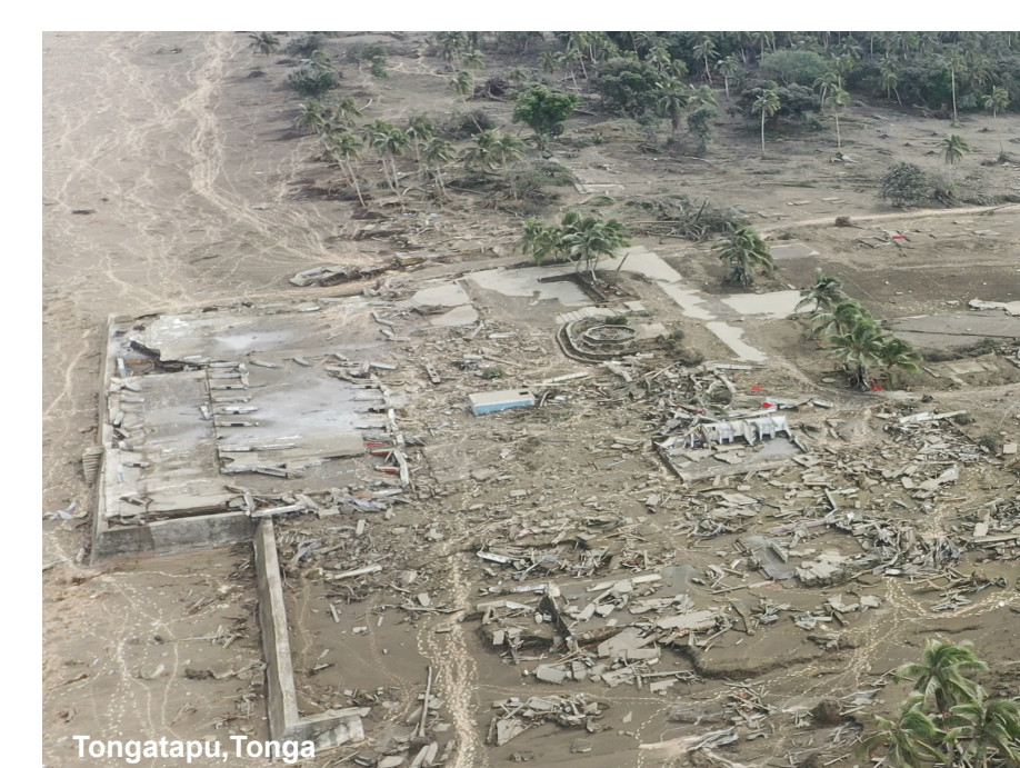
15 January 2022 tsunami. All seven resorts along the northwestern tip of Tongatapu, including the Vakaloa Beach Resort (left), were destroyed by the tsunami generated by the HTHH volcanic eruption. Credit: Tonga Geol. Svc.
