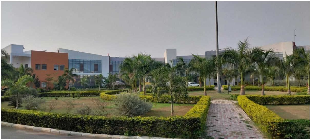
ITCOcean Admin Block - front entrance view
