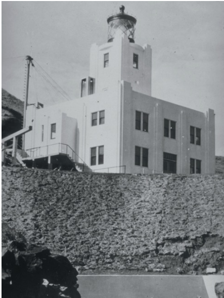
Scotch Cap Lighthouse Unimak Island
