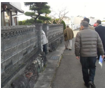
Photo 3-13 Wall of concrete block
