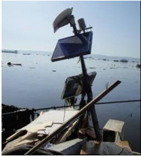
Photo 1. Damaged sea level station the day after the 27 February 2010 tsunami, Talcahuano, Chile Photo by Rodrigo Núñez Gundlach
