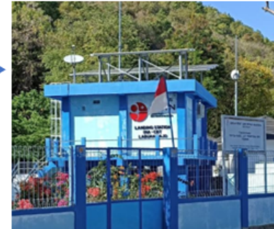
Landing Station (LS)
