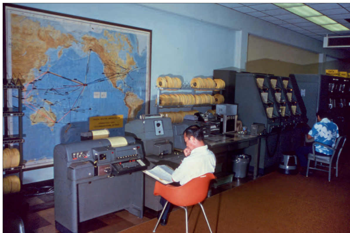
Honolulu Observatory watchstanders sitting in front of teletype machines for receiving and sending sea level readings from observing stations, circa 1960s and 1970s (Credit ITIC Archives)
