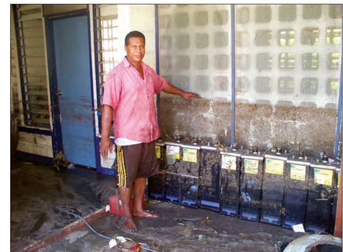
Tonga. The tsunami flooded 46% of the island of Niuauputapu. Tonga Communications Corporation services went down as waves slammed debris into the communications satellite dish and solar power panels. In the office, tsunami flow depths reached 1-2 m shorting out instrument racks, routers, and batteries. (Credit: courtesy Tonga Met Svc)
