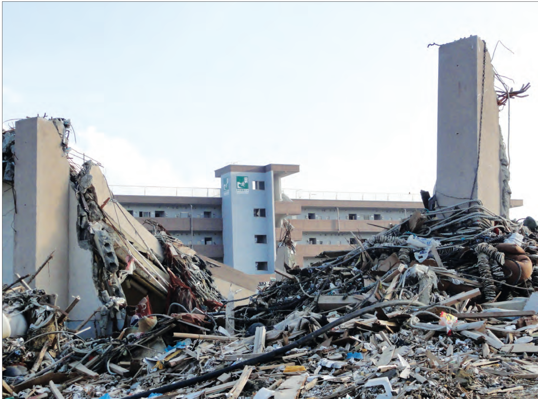
In many places, Buildings designated as evacuation shelters (green sign) withstood the tsunami waters. In Minimisanriku, the rooftop escape was needed as the waves reached the fifth (top) floor. (Credit, ITIC)
