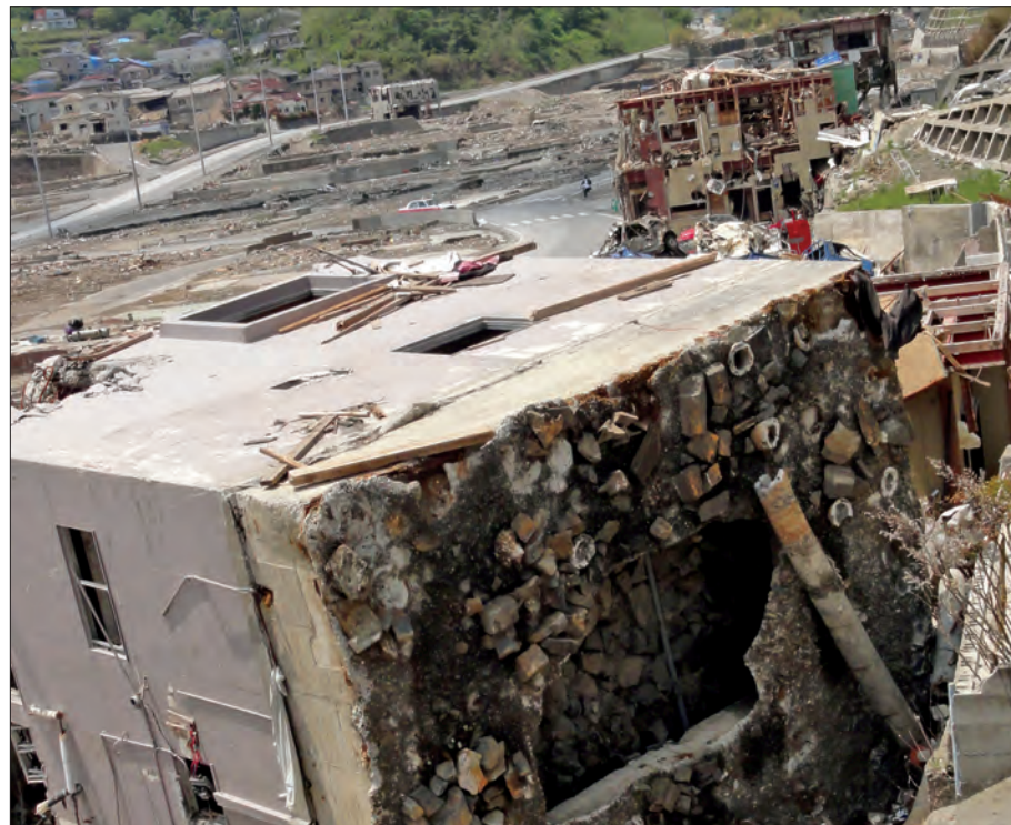
Along much of the northern Tohoku coast, tsunami flow depths of 10-20 meters were observed. (Top) In Otsuchi, tsunami waters left a yacht atop a 2-story home. (Credit: Y. Fujii, IISEE). (Bottom) In Onagawa, strong and high tsunami waves uprooted an entire 3-story concrete buildings. (Credit: ITIC)
