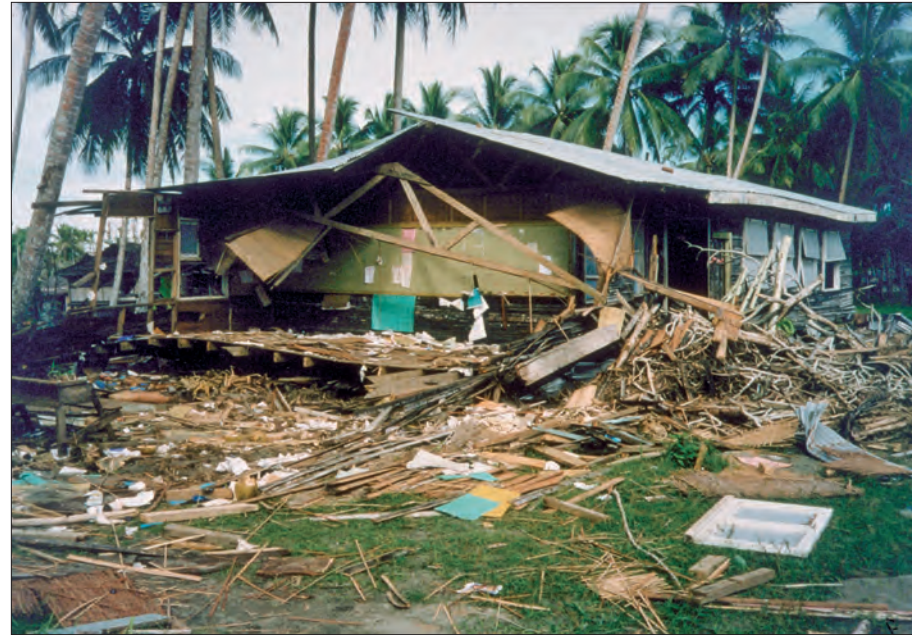
A two-story wooden school building that stood near the church at Sissano Mission was carried 65 m by the wave until caught by a grove of coconut palms. The lower floor of the building collapsed, but the upper floor class rooms were preserved. Schoolwork was still hanging on the wall. (Credit: H. Davies, Univ. of PNG)
