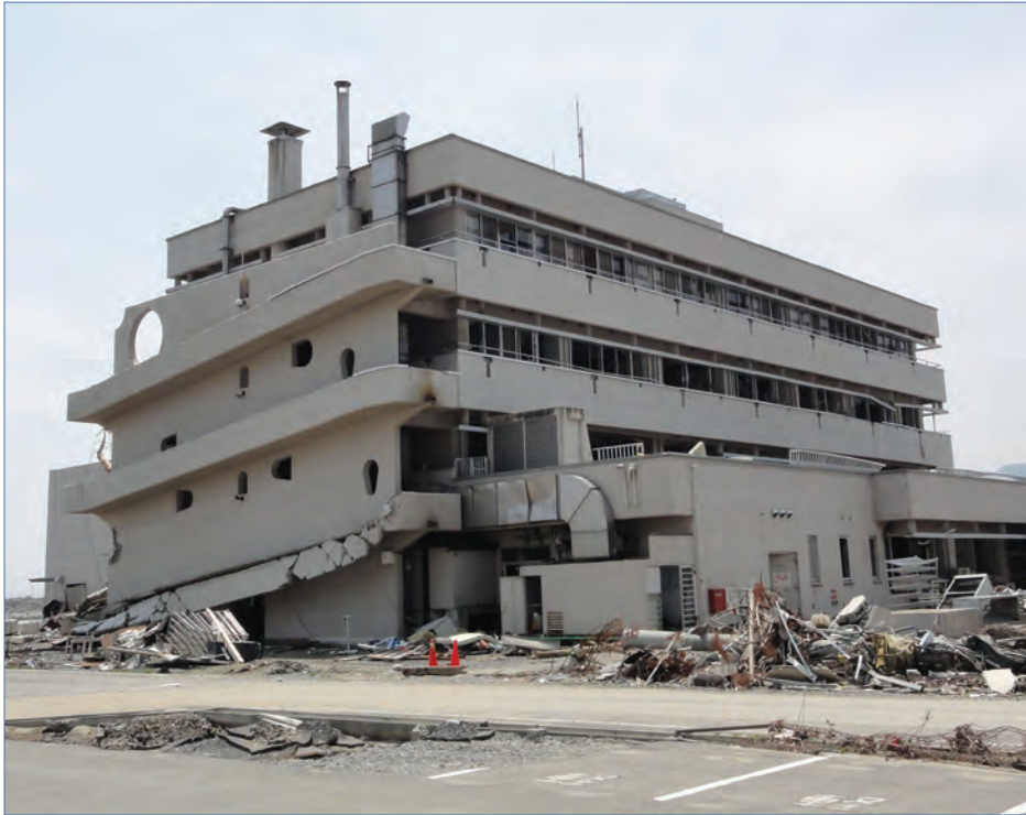
Many hospitals structures survived the 2011 Japan tsunami, including one in Rikuzentakata which was equipped with an external rampway to help people escape, and one in Minamisanriku, where external walls had been seismically-retrofit with steel braces. In both locations, the water level reached the third floor or slightly higher. (Credit: ITIC, L. Dengler, Humboldt State Univ)
