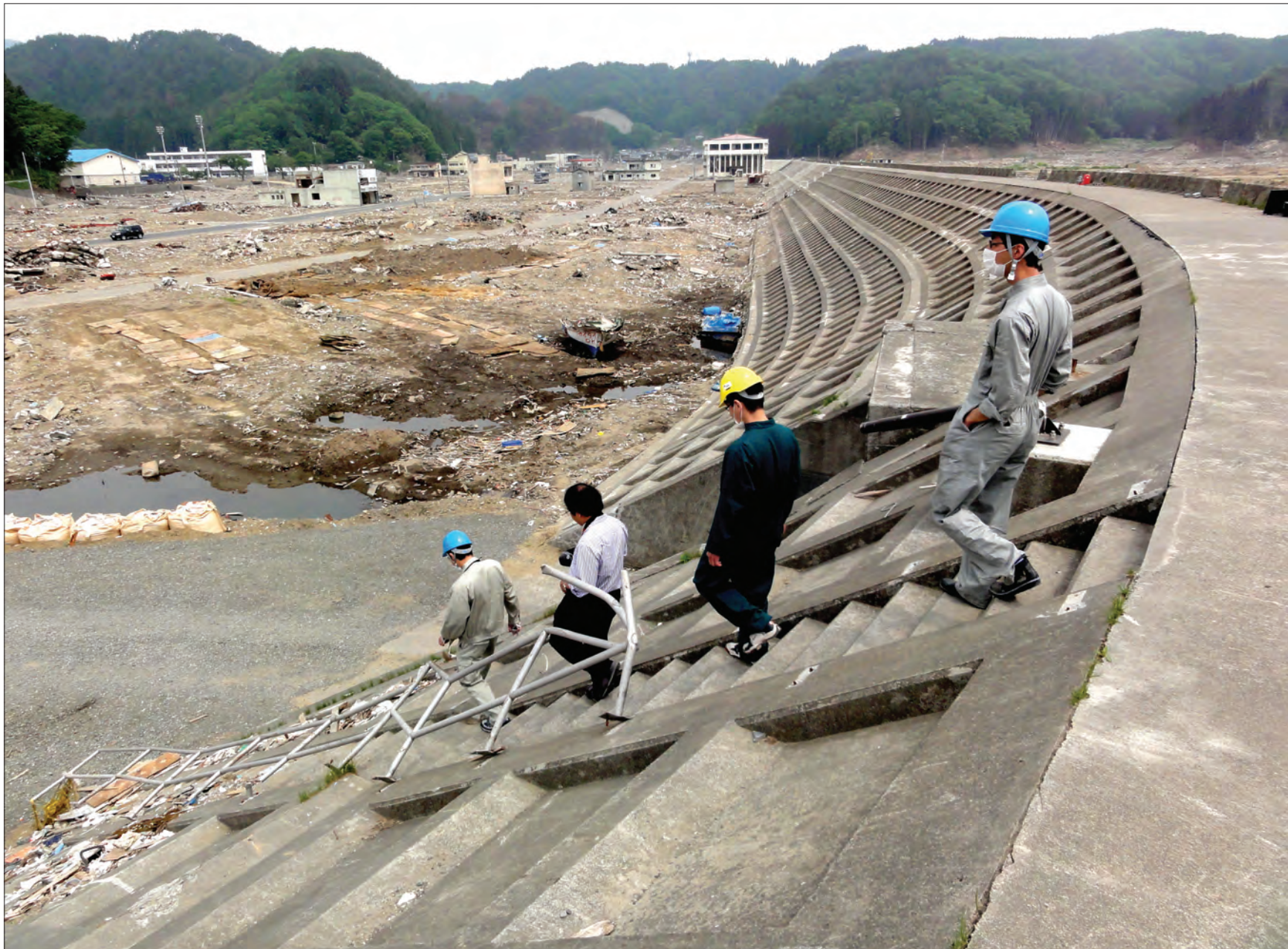
In many places, sea walls were overtopped during the 2011 Japan tsunami. In Taro, while the great wall remained mostly intact, the town behind the wall was completely destroyed as the turbulent water was unable to drain. (Credit: ITIC)
