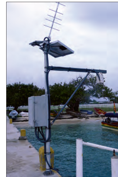
Sea level stations in Kanton, Kiribati (top), and El Porvenir, Panama (bottom). (Credit: Univ of Hawaii Sea Level Center)
