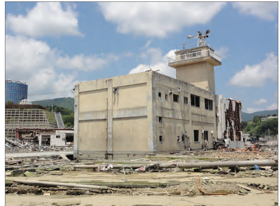
Siren and loudspeaker atop the fire station at Onagawa port that continuously alerted the townspeople of the tsunami warning; both sound and voice were used. On the left background are stairs leading to the hospital on high ground that was only briefly flooded. Despite 15-m water flow depths and velocities more than 6 m/s, the fire station survived but many low-story buildings in the town did not, with at least six buildings overturned and washed away. (Credit: ITIC)
