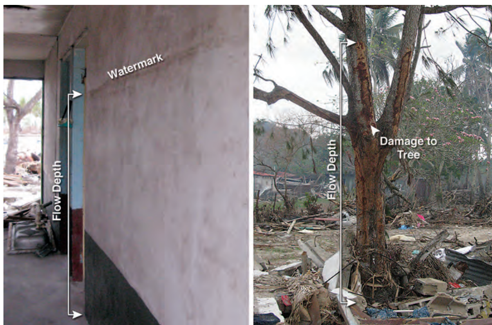
Figure 15. Examples of flow depths indicators. Left photo, below, shows a watermark within a house at Hihifo. Right photo, below, shows gouge marks and bark stripped from a tree trunk in Hihifo village.
