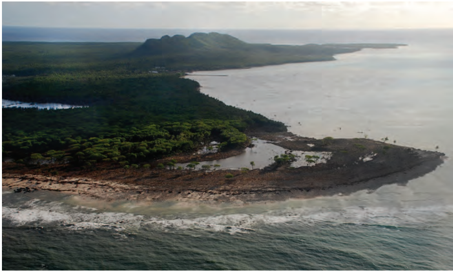
Figure 8. Niuatoputapu. Aerial reconnaissance of tsunami damage, 30 September 2009. View off northern peninsula.
