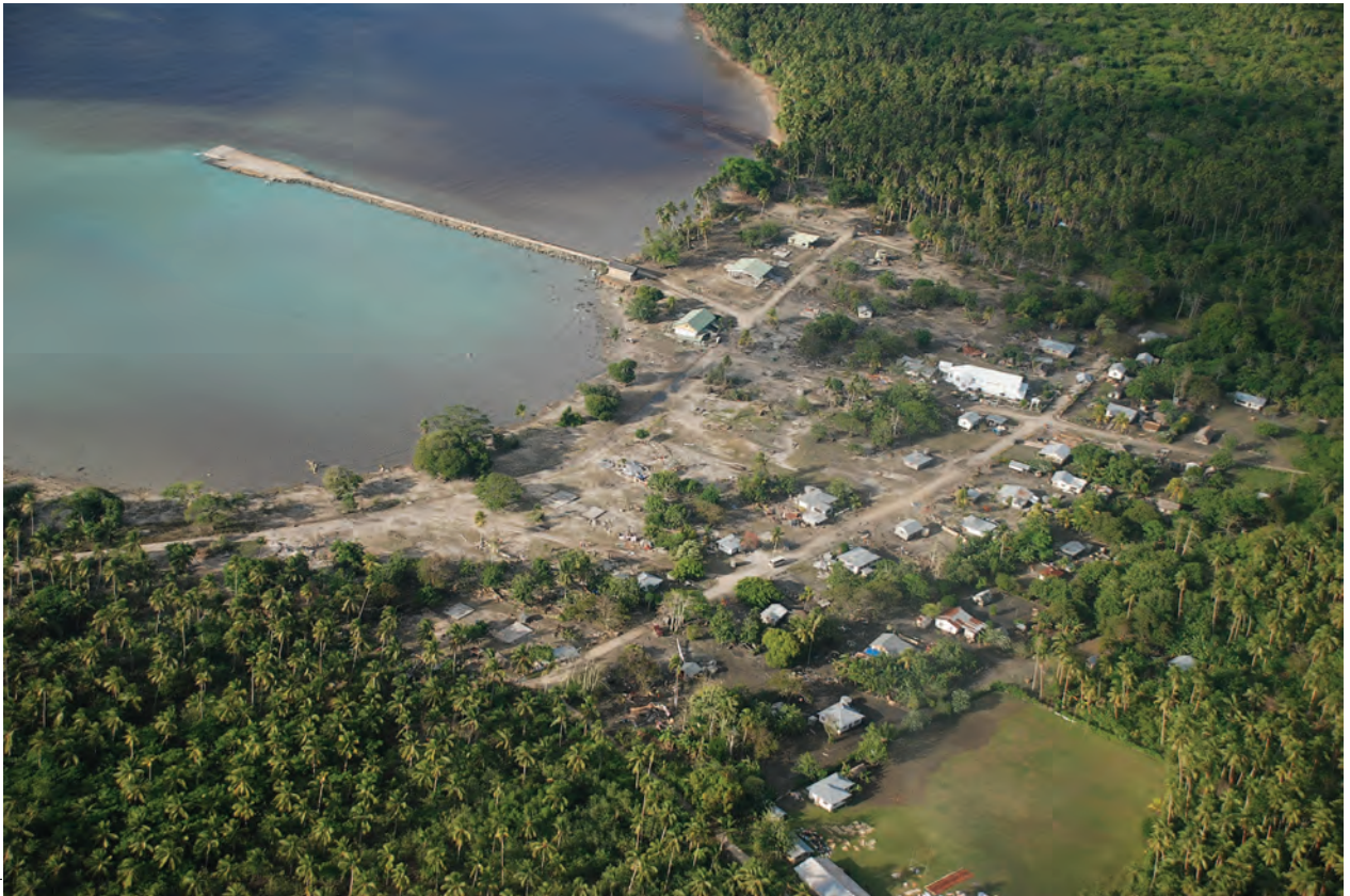
Figure 11. Falehau village, Niutopotapu. Mud spills into the lagoon, seafront homes have disappeared; and a dark stain on the school playing field (foreground in picture), marks the tsunami inundation limit. Aerial reconnaissance, 30 September 2009.
