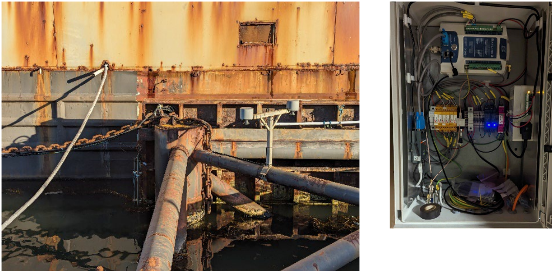
Figure 6. The repaired site at Port Stanley
