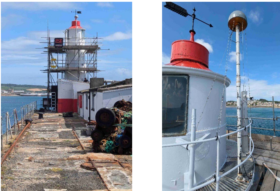
Figure 4. The Newlyn lighthouse and new GNSS antenna
