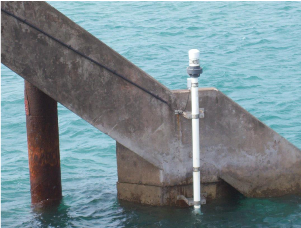
Fig 5b: The stilling well of the tide gauge at Wasini Island.
