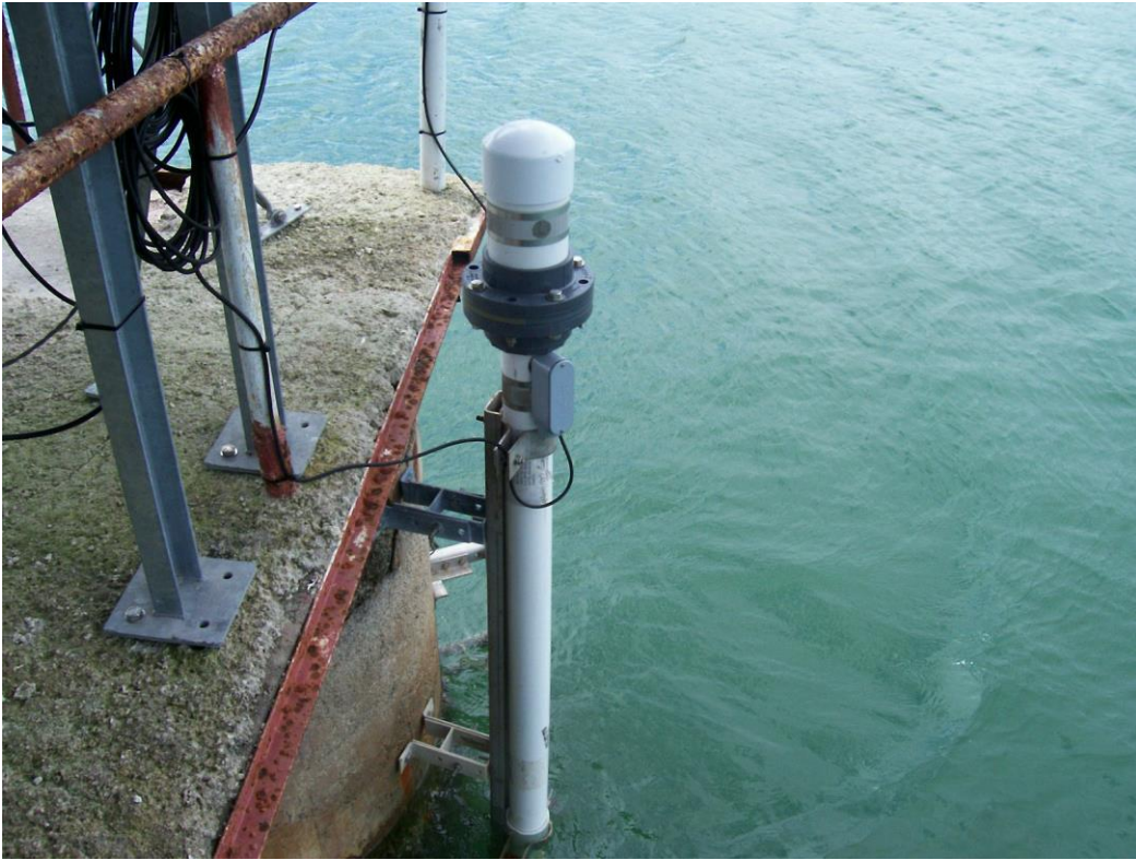
Fig 4a: Stilling well of the tide gauge at the Old Jetty of Kilifi Mnarani club.
