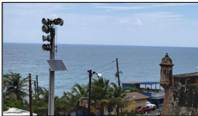
Figure. Example of coastal fixed siren installed at San Juan, Puerto Rico.
