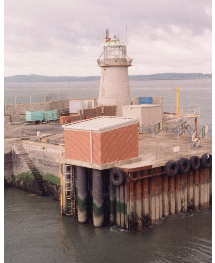
Two Stilling Wells with Float Gauges at Holyhead, UK
