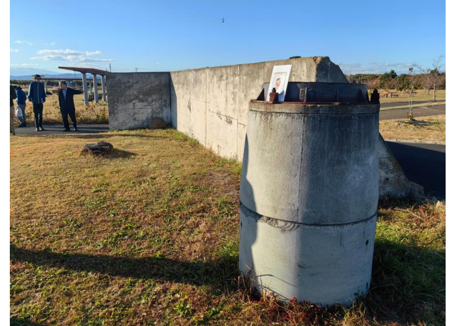
Manhole lifted by buoyant force
