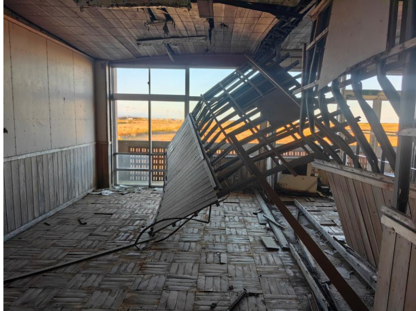
Damaged partition
