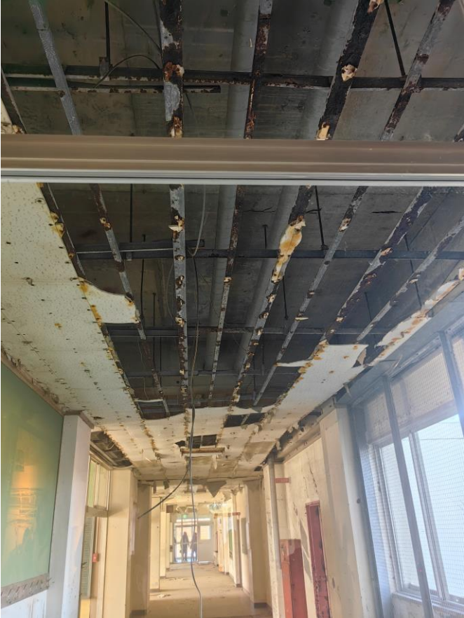
Damaged Ceiling
