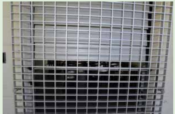
Figure 3-10. This screen at the Marshall Islands Middle School is made of strong aluminum bars in both directions and is attached to the CMU or concrete walls with embedded anchor bolts. The louver behind the screen can still be struck by small flying gravel, so should be made of shatterproof glass, glass with protective laminate, or aluminum slats for additional safety for those inside.
