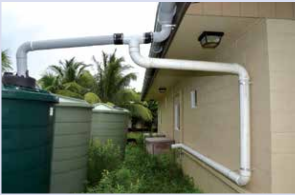
Figure 4-52. First-flush systems help to keep your water catchment system clean and reduce the need for maintenance. Dust, debris, or fecal matter that collects on your roof is washed off when it begins to rain and collects in the diversion pipe to the right. After a sufficient amount of rain has washed the roof, and the diversion pipe is full, either a pipe bend or a floating ball valve diverts water to the left where it is collected in the water tank.
