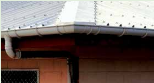
Figure 3-6. Marshall Islands High School has many of the criteria looked for in a shelter. Note corrugated metal roof with sufficient fasteners and large washers to hold the metal roofing down during high wind events. The fasteners should be ring-shank nails or screws that are well-embedded into the supporting roof trusses, rafters, or purlins.
