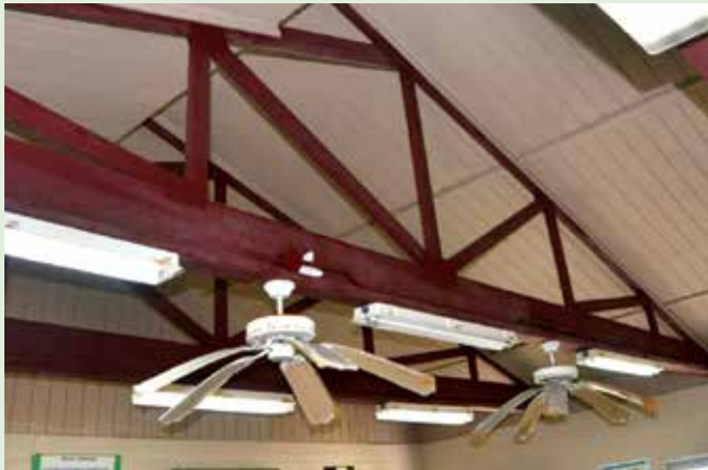
Figure 3-7. The roof trusses should be engineered and pre-manufactured. This will be standard in newer government buildings, especially schools. It will not be for older buildings. This photo shows a typical roof truss at Marshall Islands High School.
