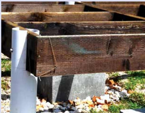
Figure 4-36. Example of ACZA wood suitable for use in the marine environment. Note the cuts or incisions on the surface to increase penetration of the chemical treatment. Because the chemicals in this wood are very corrosive, as well as the marine environment itself, stainless steel fasteners are used to attach the column to the wood joists (support for the flooring). Photo courtesy of Ben Chutaro.
