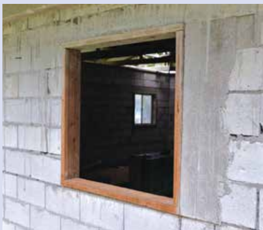
Figure 4-29. Typical window for a concrete house in Majuro has the window framed by 2 inch by 4 inch, or 2 inch by 6 inch termite treated lumber. If the window framing and concrete wall are flush, plywood can be cut to overlap the treated framing lumber by 1 or 2 inches. Then fastener holes can be pre-drilled in the plywood at a pre-determined spacing to hit the middle of the 2 inch by 4 inch or 2 inch by 6 inch, while staying away from the edge of the plywood. If the window framing is inset, the plywood must be precisely cut to insert in the inset. Fastener holes should still be pre-drilled into the plywood.
