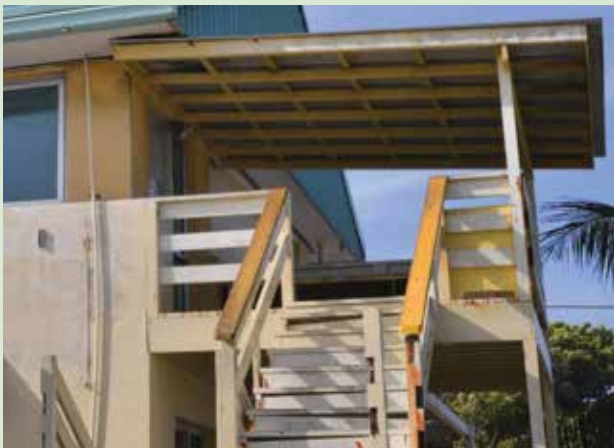
Figure 3-13. Some sturdy reinforced-concrete buildings have wood stairs to the second floor. They are likely to be damaged or washed away during heavy wave inundation. Such contingencies need to be planned for by having an emergency ladder readily accessible on the second floor. Note that the roof over this upper landing is also likely to be damaged or blown away during a typhoon. Photo of the Majuro Youth Center.
