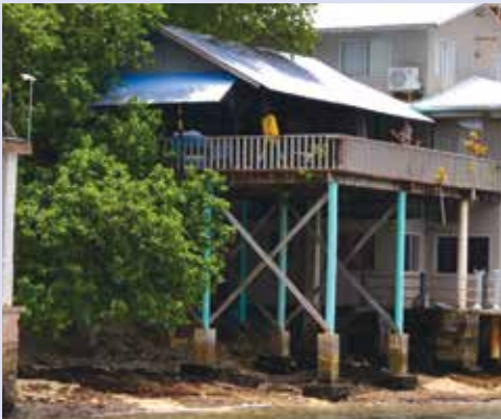
Figure 4-40. This house in Majuro was elevated to prevent damage from wave inundation and flooding. This is an extreme example of elevation of structures. Many houses in Majuro have been elevated a more modest amount (see Figure 4-41). This house has a spread concrete footing (see Figure 4-42). The brown wood members forming the X pattern are cross bracing to provide additional lateral support of the structure.
