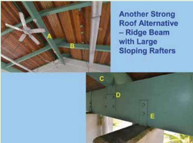
Figure 3-8. Another strong roof design is to have a ridge beam (A) attached with steel connectors to large sloping rafters (B) (top left photo). The sloping rafter (C) then connects to a horizontal beam (D) with a steel plate (bottom right photo). The beam is connected to the concrete column (E) with another steel connector. Photo from Marshall Islands Middle School.
