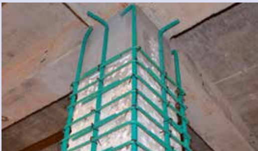
Figure 4-47. Example of epoxy coated rebar about to be encased in concrete. Any bends or cuts in the rebar that cause the epoxy to come off should be recoated.
