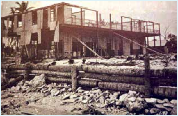
Figure 2-6. Typhoon Wind Impacts - Damage to the Catholic Girl's and Nuns' Living Quarters building in Jaluit after the 1905 typhoon. Note the blown off roof, which is common from the strong winds of a typhoon. In addition, there is water damage or inundation that overtopped the log seawall and eroded or scoured sediment behind the wall (Photo Micronesian Area Research Center).
