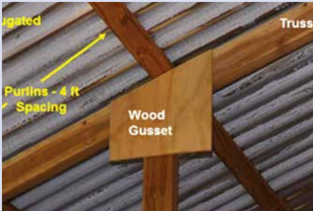
Figure 4-17. In an enlargement of Figure 4-15, on top of the trusses, are wood purlins (2 by 3's) running perpendicular to the trusses and parallel to the length of the house. The metal corrugated roof is attached to the purlins. It is important that the purlins are strongly fastened to the trusses. This can be done for new buildings and in retrofit, if a ceiling does not cover the roof structure.
